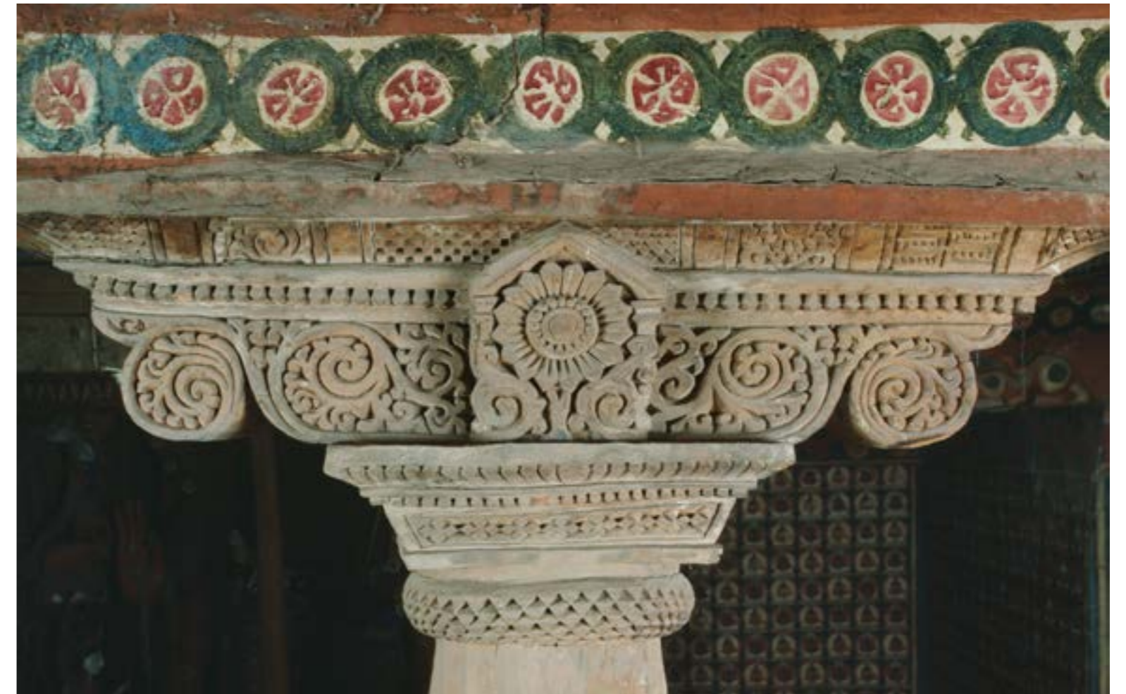
516 The 'Ionian' capitals crowning the grooved columns in the same building, with their volutes at both ends, are late offsprings of Central Asian antecedents. In simpler forms, but also executed in wood, they appear already in the third century CE in Loulan and Miran, and in the sixth century in Khadalik. Their models may perhaps be sought in Persepolis or even further to the west in the Mediterranean area, with intermediate stages in Taxila, Gandhāra. The scroll-work carved into the Alchi capitals is directly derived from similar elements in Kashmiri masonry decoration.
