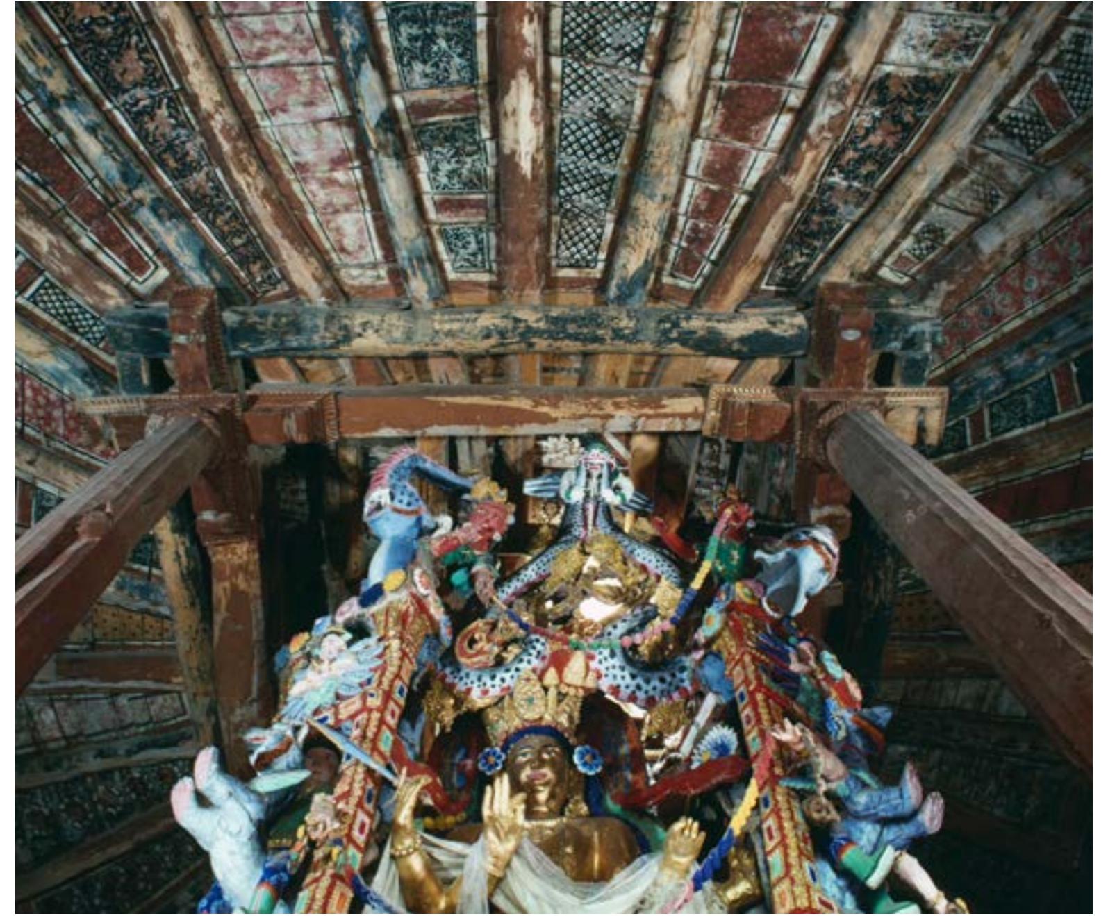
264 Entering the temple in front of the golden Mañjuśrī and looking upwards offers a perfect view on the unusual ceiling construction, with the spaces between radiating cross-beams filled with a rich array of textile patterns. From this side a roughly symmetrical distribution of these patterns can be noticed.
