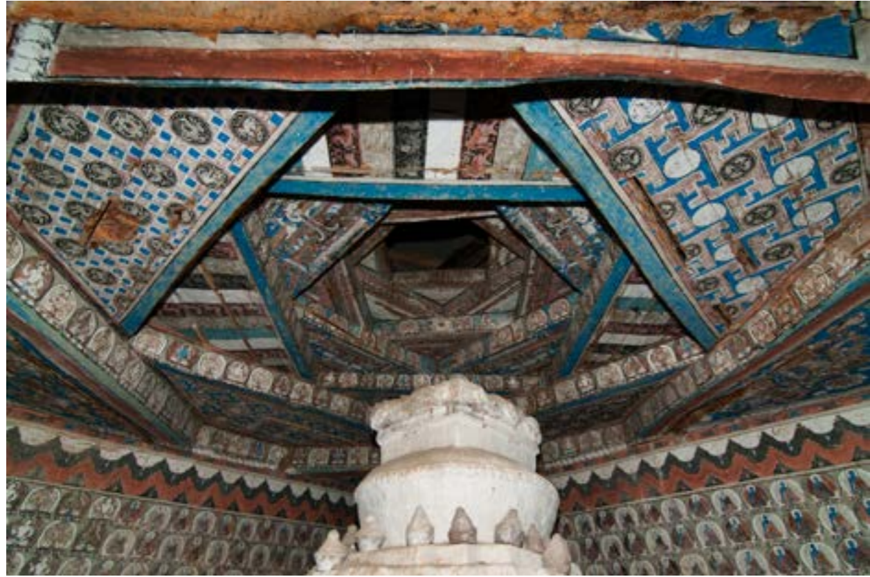
348 Of the eight layers of the lantern ceiling of the Palden Drepung Chörten the top panel is lost. It must have contained an image of Mahāvairocana. CL 2010 (5879).
